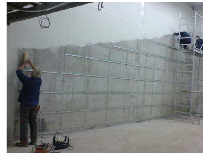
Fixing of Rails
