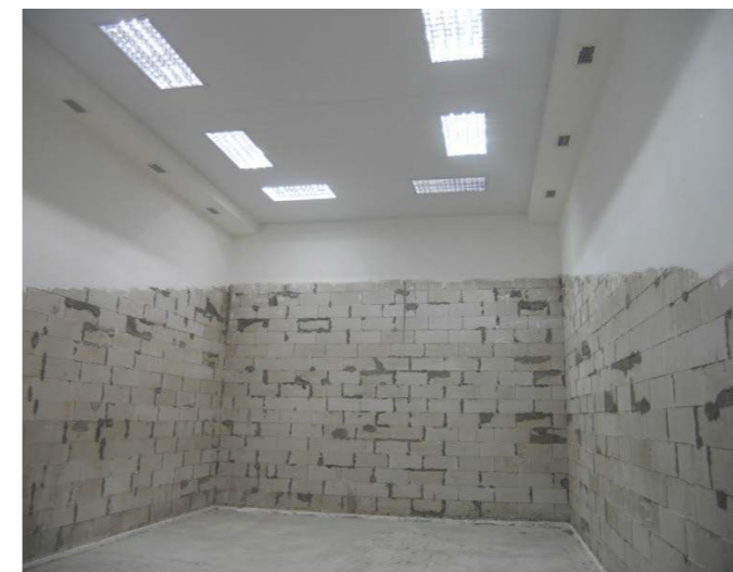
Before start of installation
