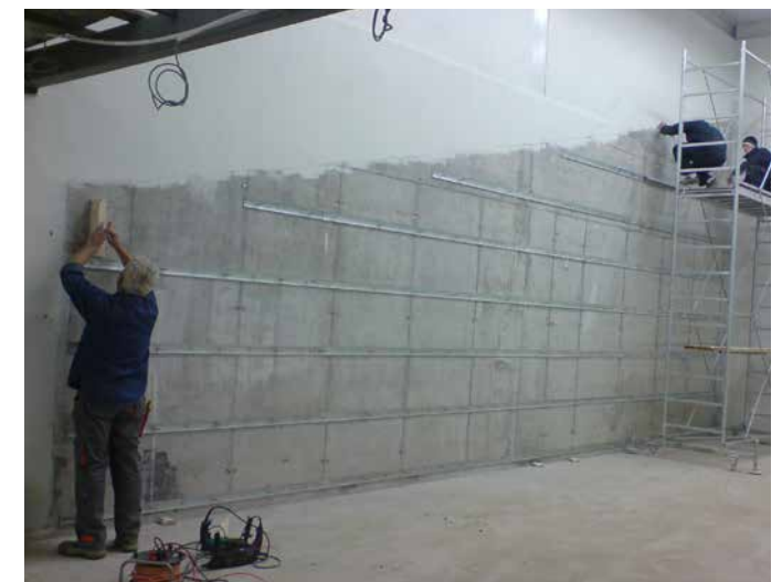
Fixing of Rails
