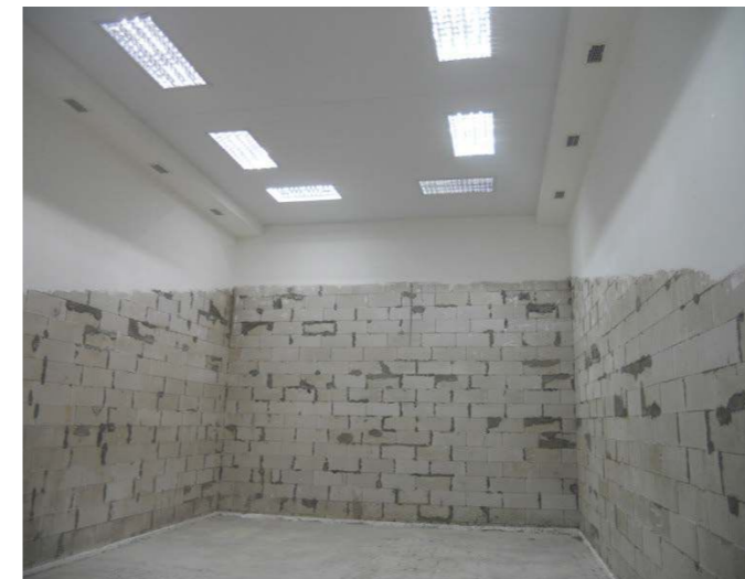
Before start of installation
