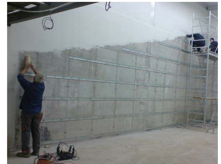
Fixing of Rails
