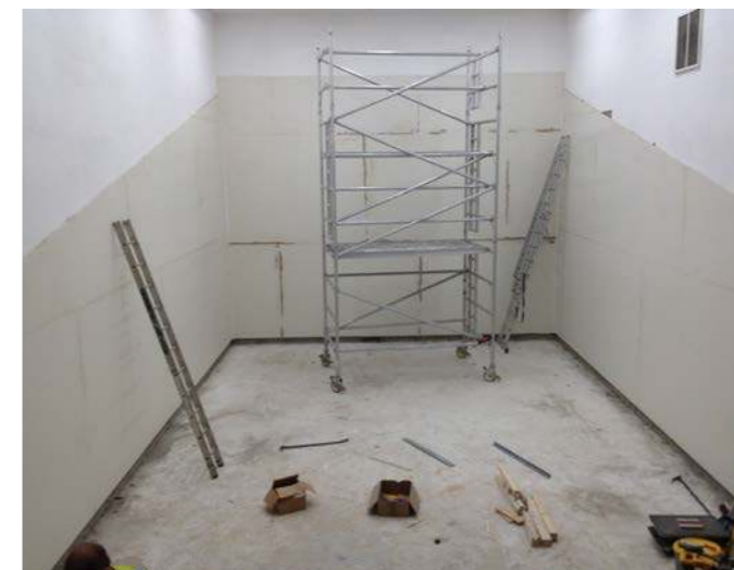
Before final coating
