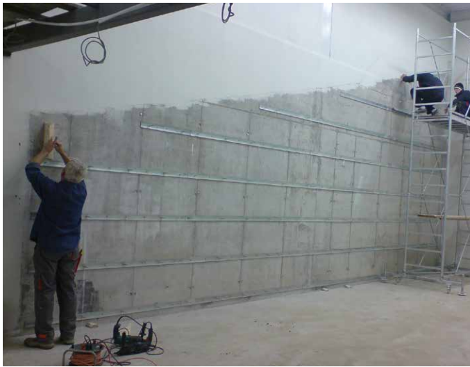
Fixing of Rails
